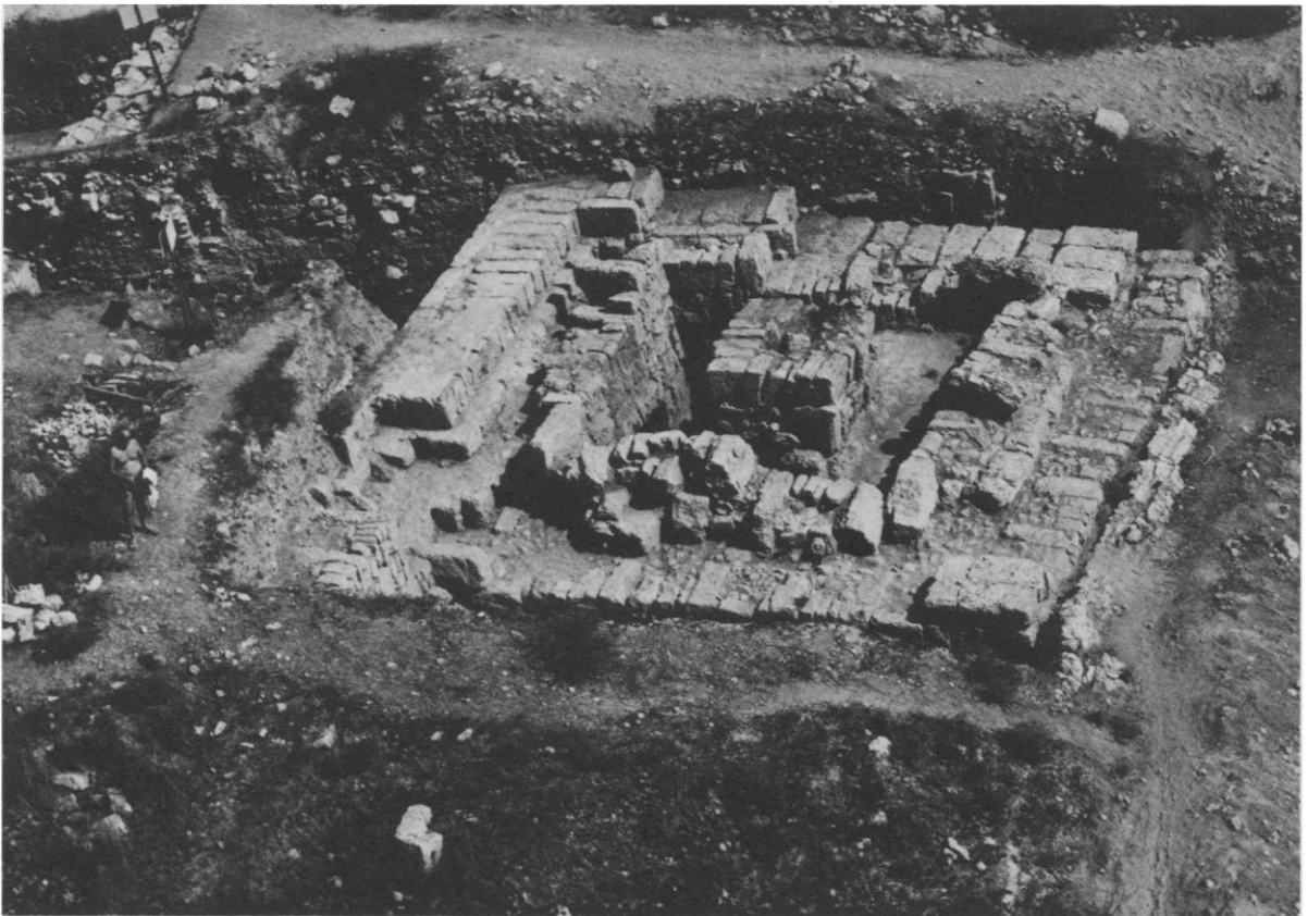
Fig. 5. Tel Dor, Hellenistic city wall and tower in Area A. Headers-against-a-stretcher pattern is seen at the back of the tower, headers-out in the central pilaster. The foundations are constructed in the compartment building technique; note the “diatons”—large headers projecting from both faces into the rubble fill, dividing it into a series of constructional compartments.
